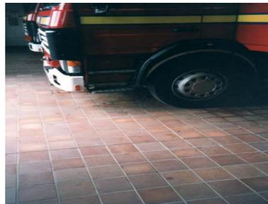
Applications where heavy-duty tiles are used successfully include factory floors, appliance bays in fire stations, loading bays in warehouses and motor vehicle workshops. Heavy duty slip-resistant tiles are also available and should be used in areas which are likely to be wet, trafficked by vehicles, or where increased slip resistance is required.
