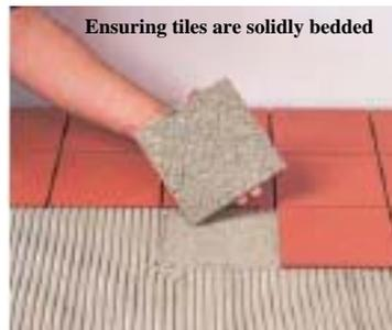
Tile spacers should not be used on natural quarry tiles and grout lines should be maintained to give a **minimum** joint width of 6mm for subsequent grouting.
