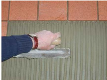
Tiles should be pressed firmly into position with a slight twisting action. It is essential to ensure each quarry tile is fixed on a solid bed and that the entire tile back is in full contact with the adhesive. Tiles should be lifted periodically as work progresses to check this. Any voids underneath tiles will be a potential point of weakness under load and in exterior situations water may accumulate giving rise to frost damage.
